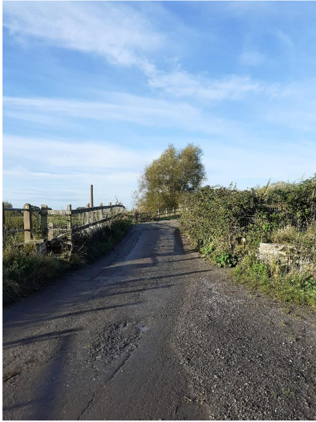
3. Point A1 facing south-west towards Long Sutton Catchwater Bridge
