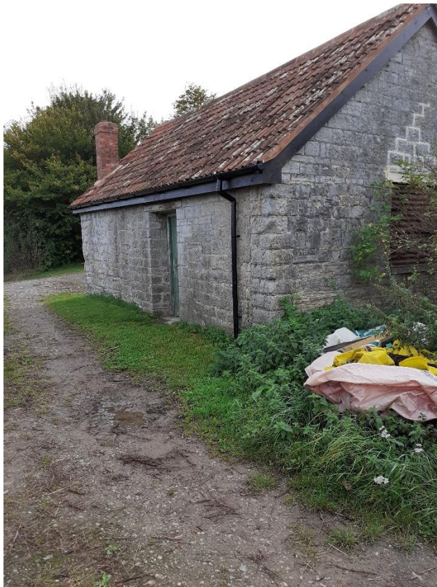
24. Lime Kiln building between points E and E1
